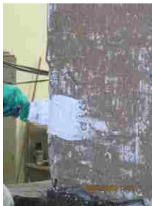
(b) Application of MBrace® Putty
