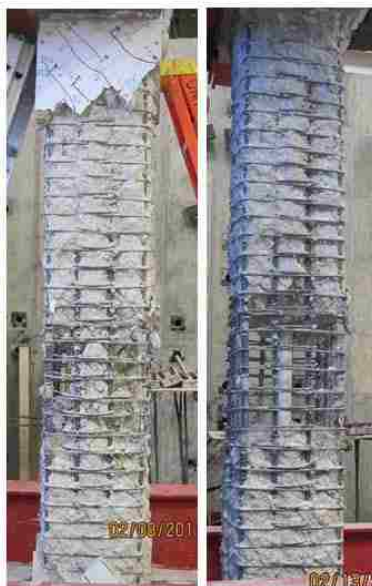
Figure A.2. Before and After Removal of Loose Concrete
