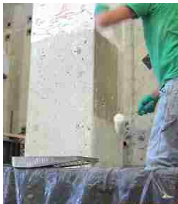
(a) Application of MBrace® Primer
