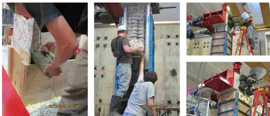
Figure A.4. Placement of Repair Mortar
