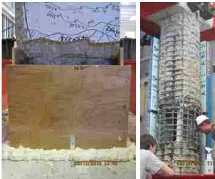
(a) Plywood Formwork
