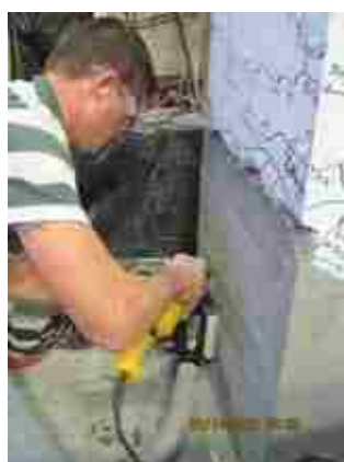
(a) Smoothing Concrete Surface
