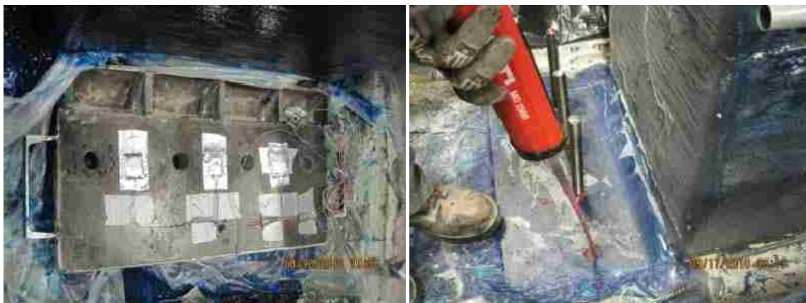
(a) Temporary Placement of Anchorage Over “Wet” Saturant
