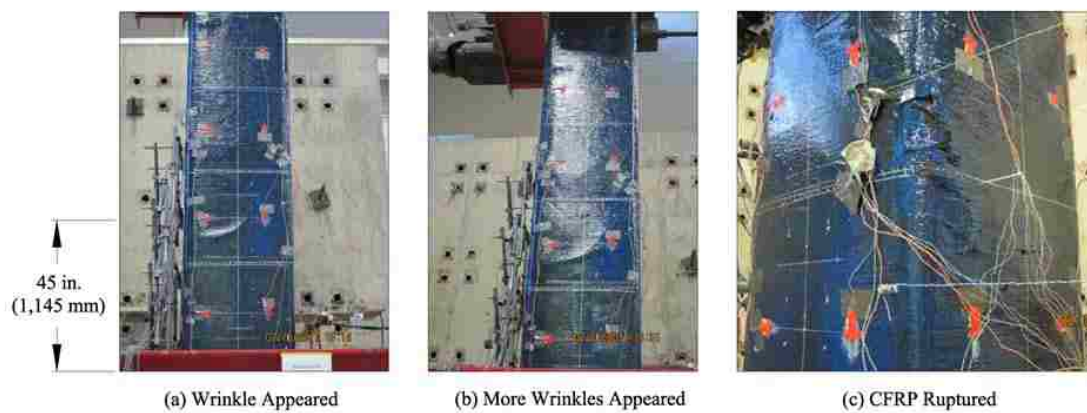
Fig. 5 - Failure of repaired column.
