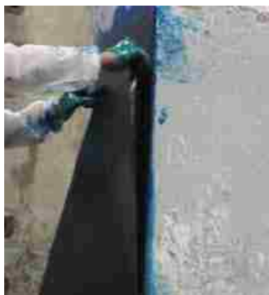
(a) Application of Longitudinal CFRP
