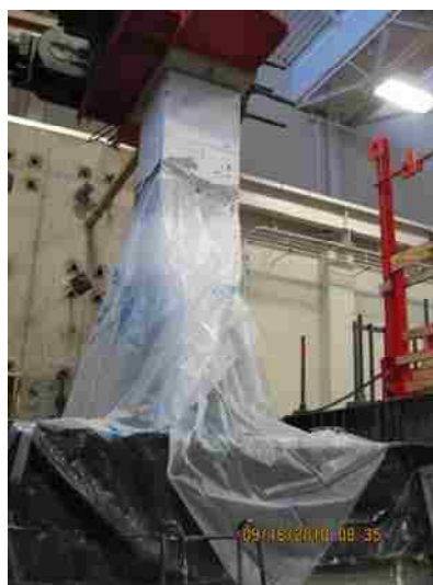
Figure A.8. Curing of the CFRP System
