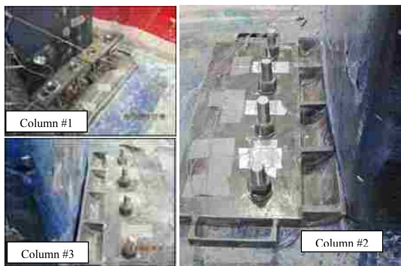
(c) Installed Novel Anchorage System
