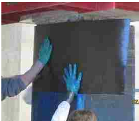
(b) Application of Transverse CFRP
